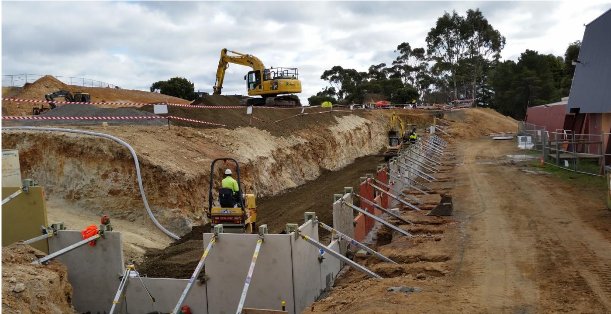
Construction of the retaining wall
