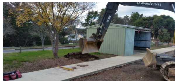
Foundation works for netball shelter.
