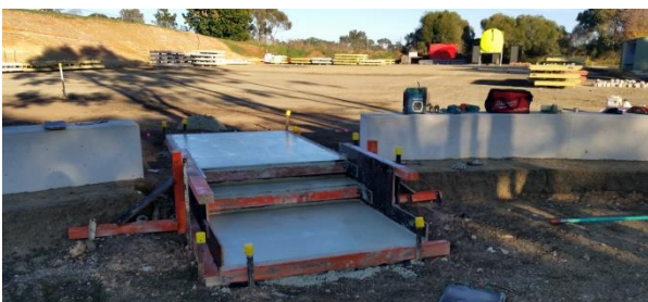
Concrete stairs and seating in forecourt.
