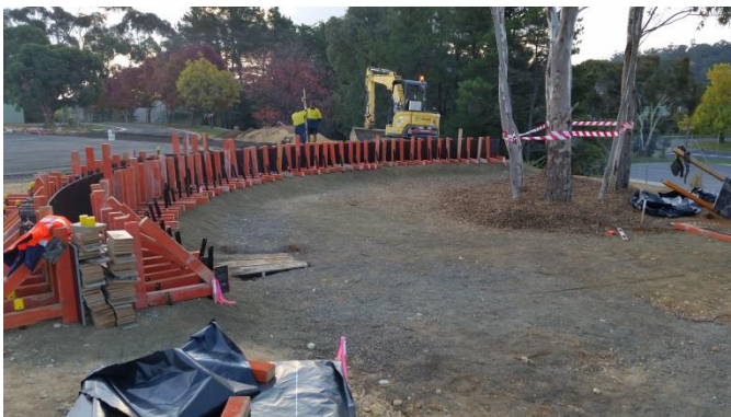
Foundations for forecourt seating
