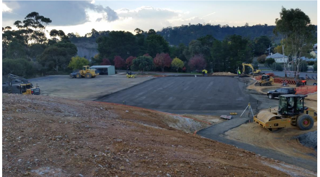
Base preparation for asphalt netball courts
