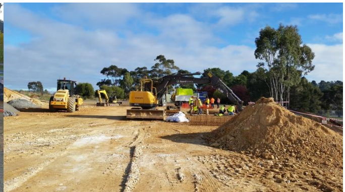
Excavation works for acrylic netball courts
