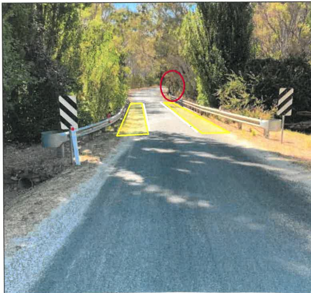
Photo 2: View to the southeast from the proposed Give Way line. Suckers to the southwest of the bridge (marked in red) require removal and trees trimming to improve the view to oncoming traffic. Also note proposed edge lines on bridge providing a single 3.5 m traffic lane and definition of non-trafficked areas with yellow cross-hatching.
