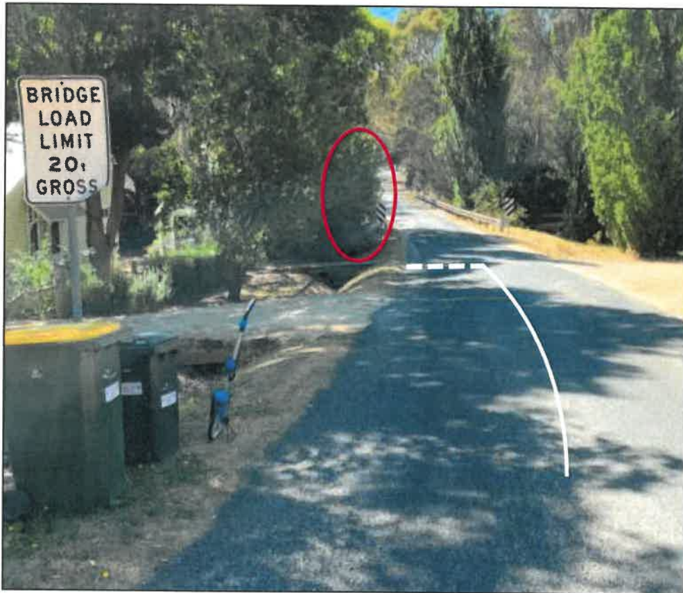
Photo 1: Trees to left of road at the northwest approach need trimming to provide a clear view to the roadway to the southeast of the bridge. Note the location of proposed Give Way markings.
