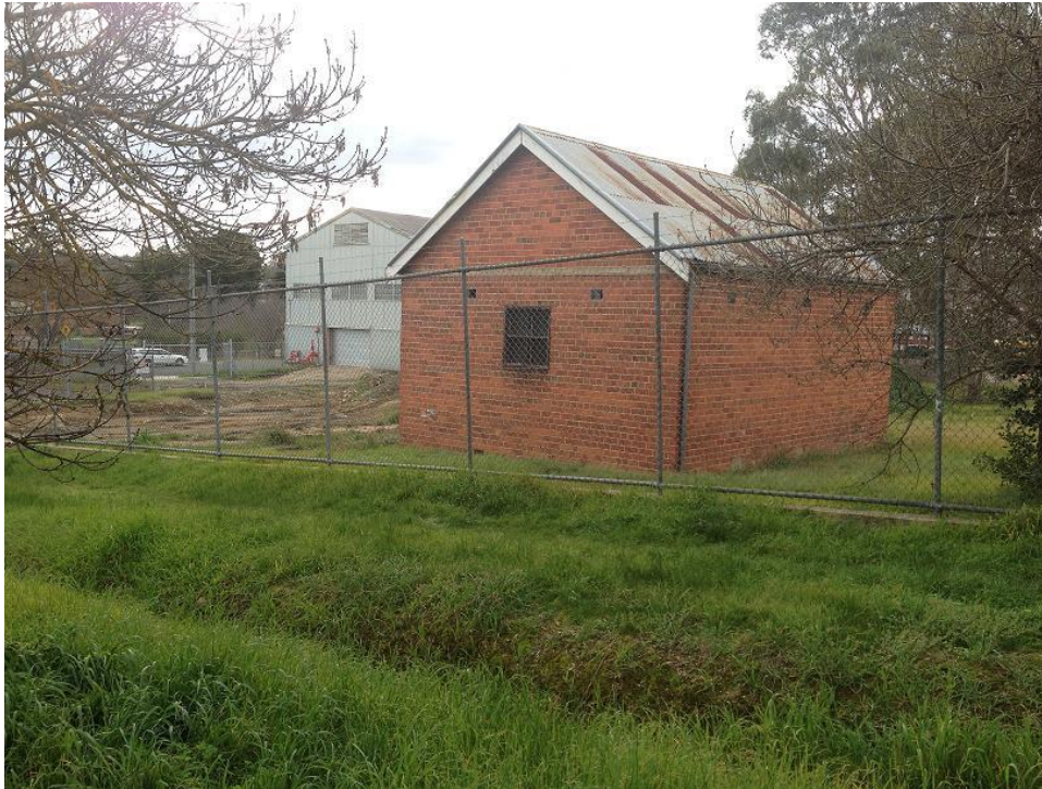
Photo 5: Brick store room at south east corner
