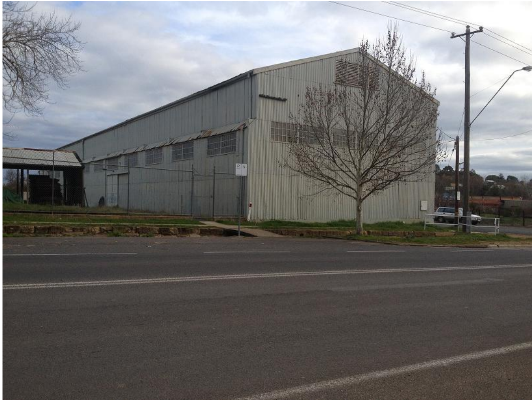
Photo 3: Portal frame shed, currently empty, on corner of Parker St and Kennedy St
